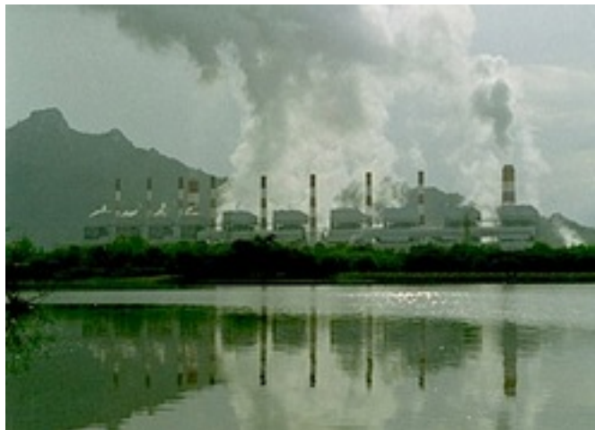
Coal Fired Power Plant
